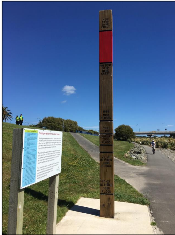
Figure 11: Flood markings pole with major floods and new stopbank height (top of red section)
