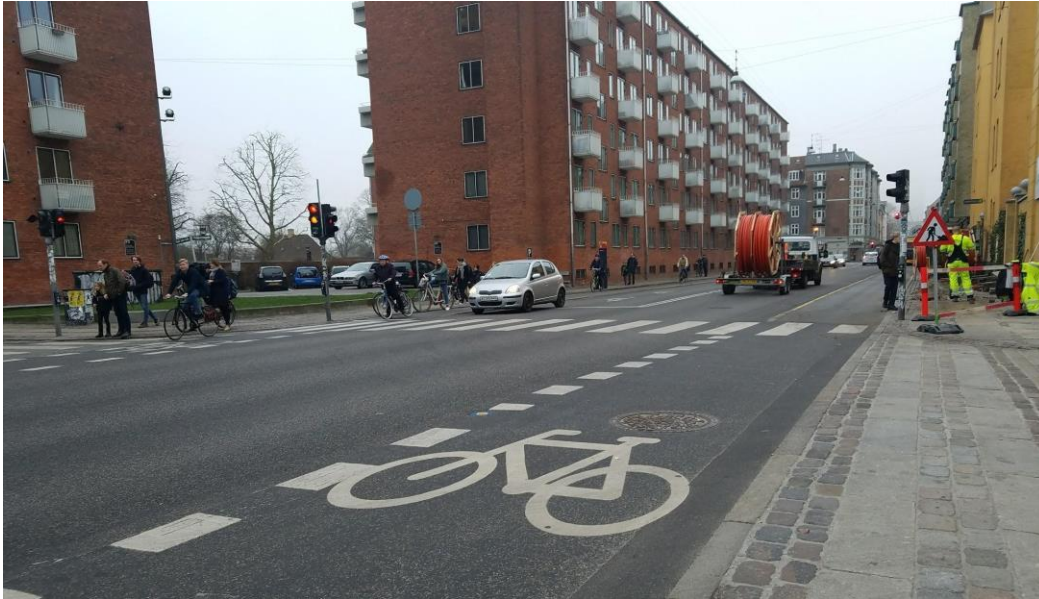
Figure 8: Road Construction on Prinsessegade
