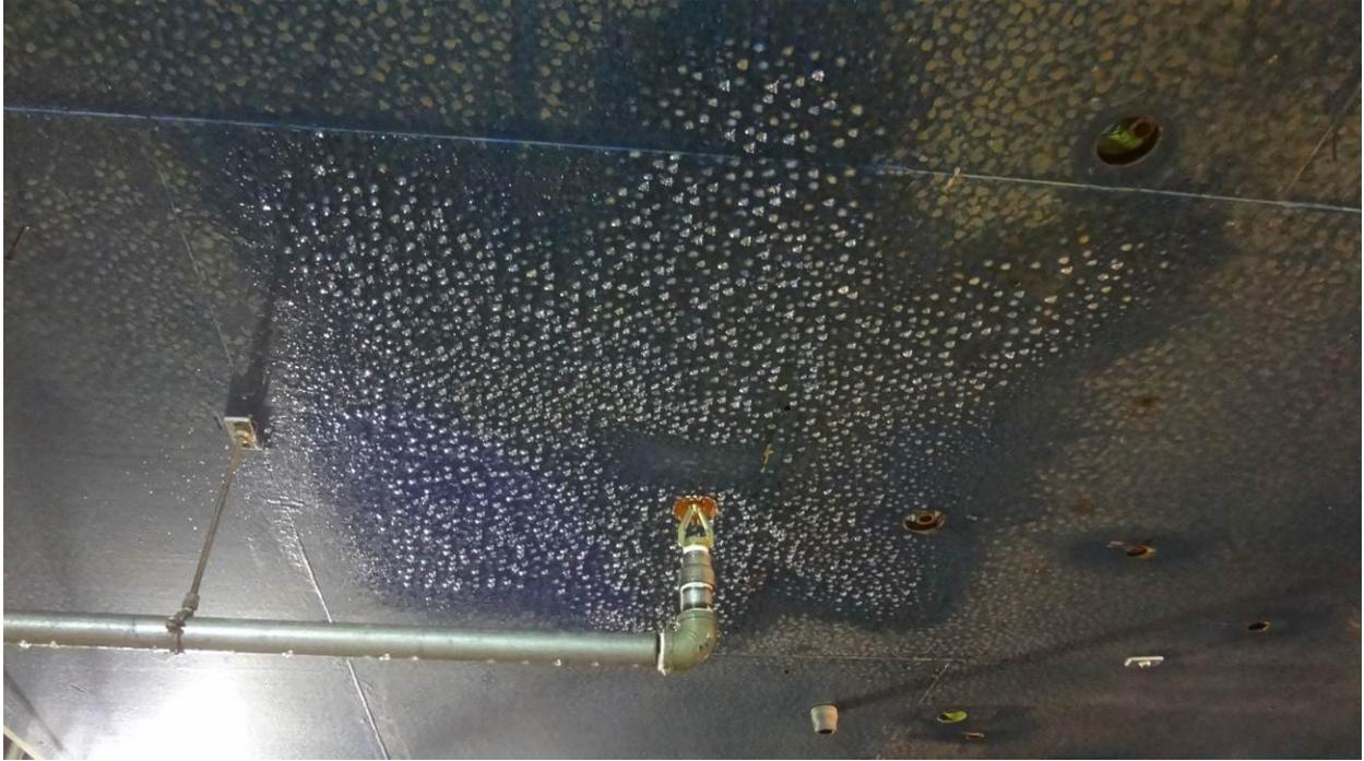
Figure 42: Droplets on Ceiling
