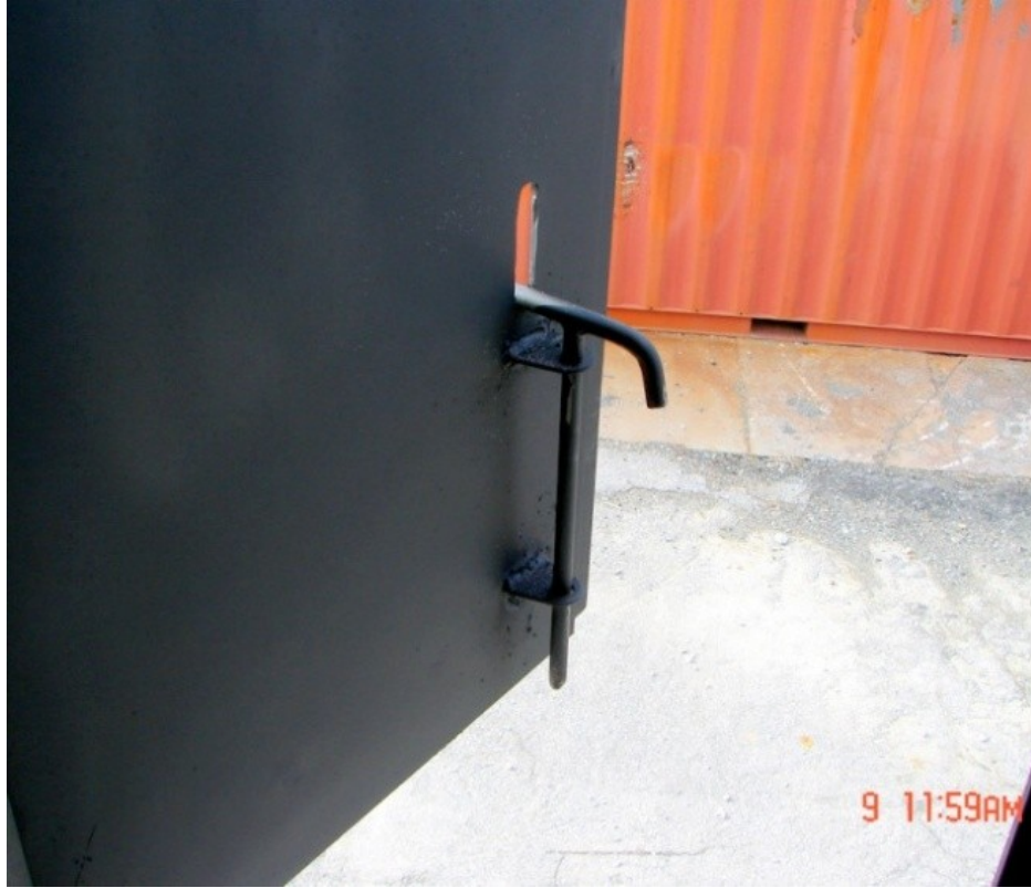
Figure 4-11: Window & Latch Construction
