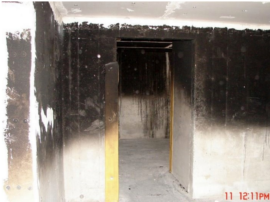
Figure 4-12: Interior view of Burn Facility
