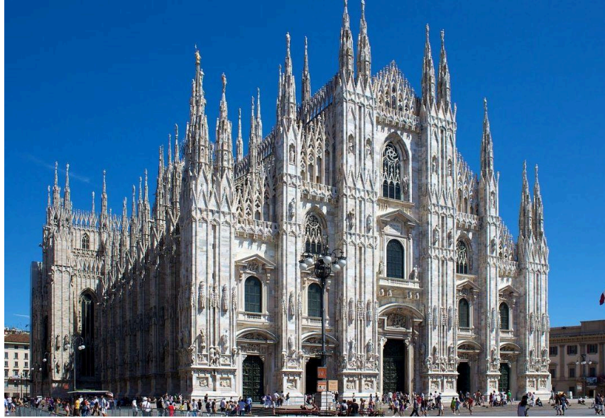
Figure 3.8 - Photo of the Milan Cathedral used for reference
