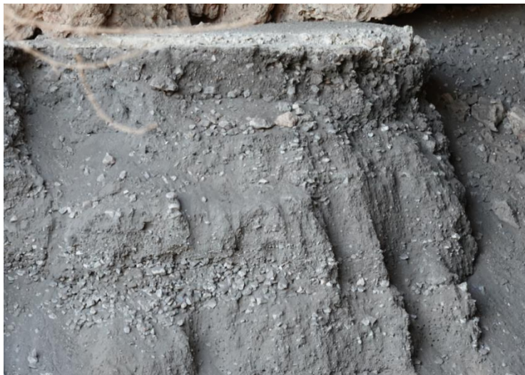
Figure 10. Top Layer of Lime Mortar on Cave Floor Filled During French Military Occupation.
