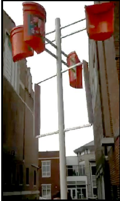
Figure 32. Completed Savonius-Darrieus wind turbine.
