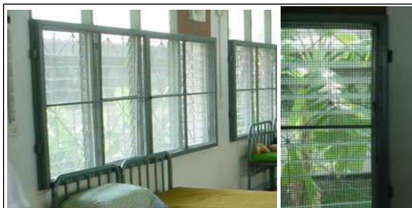
Figure 34: Protective Window Guards in Building 2
