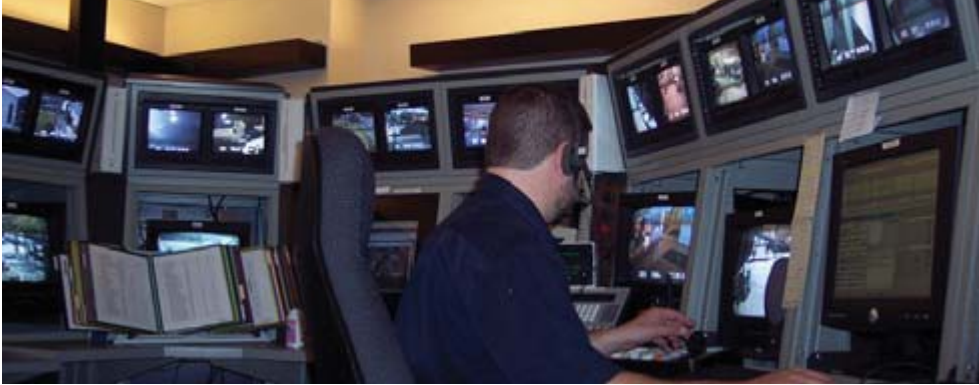
Figure 3 shows the University of Pennsylvania Control Room for CCTV.
