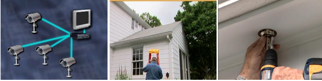
CCTV systems consist of cameras connected to digital video recorders, which are connected to monitors. Mounting bracket is screwed into place under the eave of the house.
