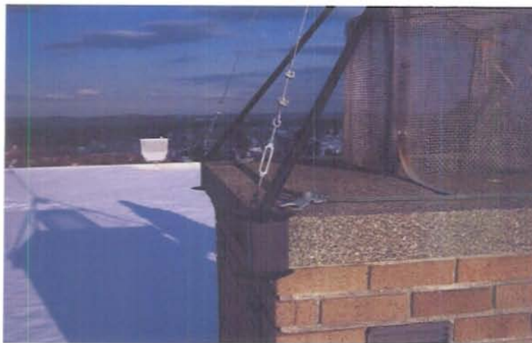
Figure 33: Guy Wire Turnbuckle Connection
