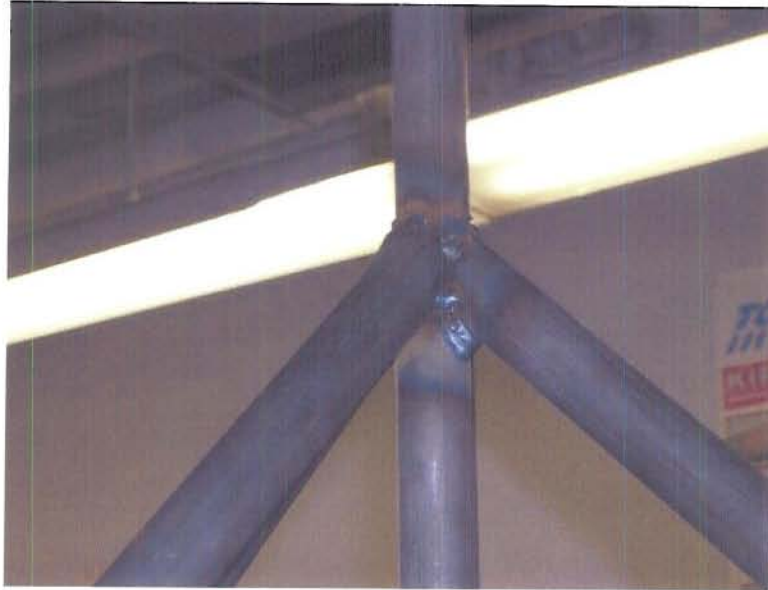
Figure 27: Close Up of Supporting Pole Connection
