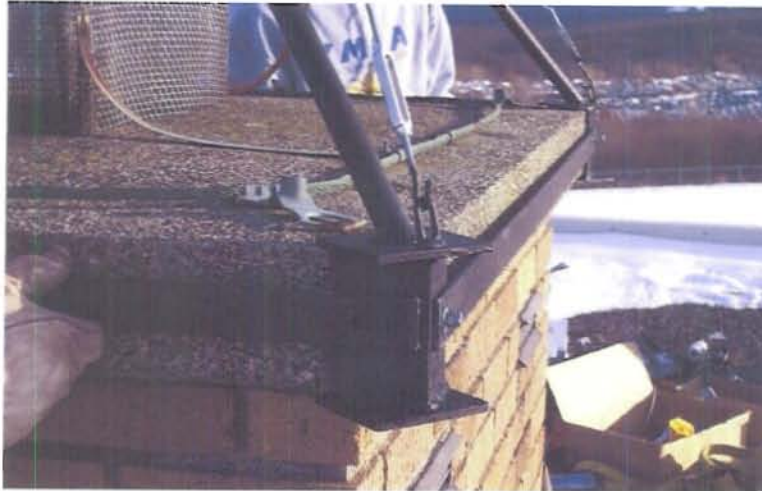
Figure 32: Corner Bracket and Braces Being Installed
