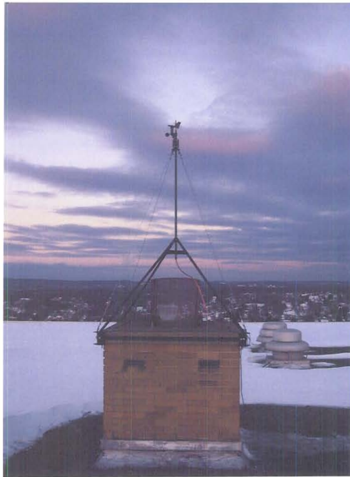
Figure 35: Tower Fully Installed
