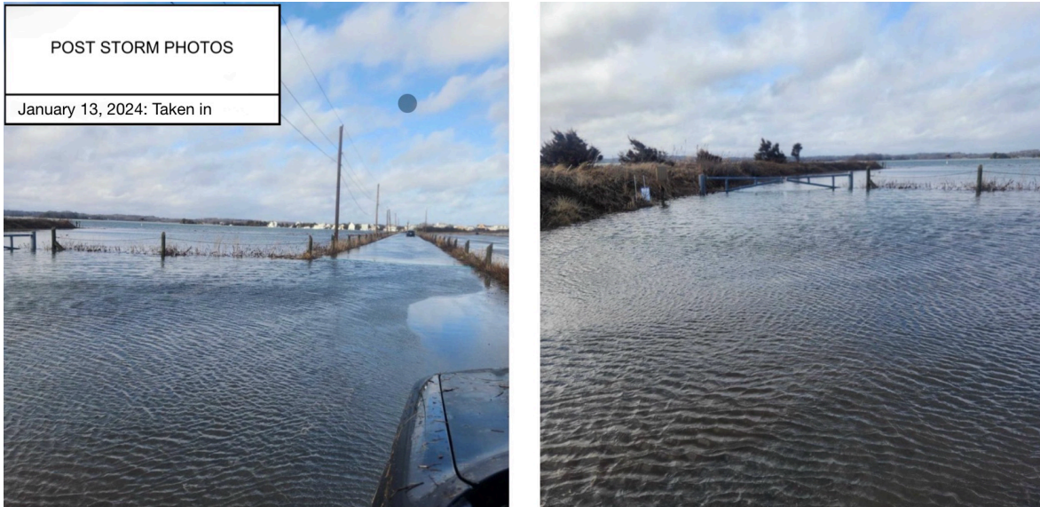
Figure 10: Image of flooded Duxbury Parking lot post-storm surge.
