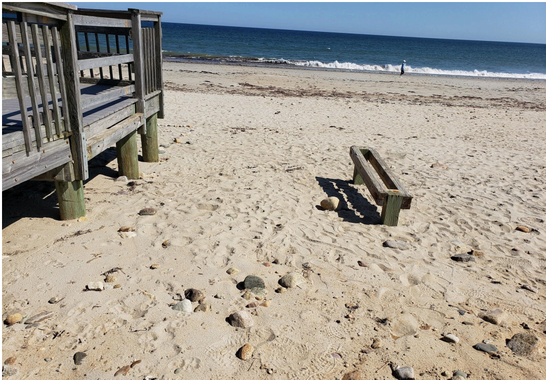
Figure 12: Shows the ocean-side ramp of the Duxbury Beach Parking Lot Boardwalk removed
