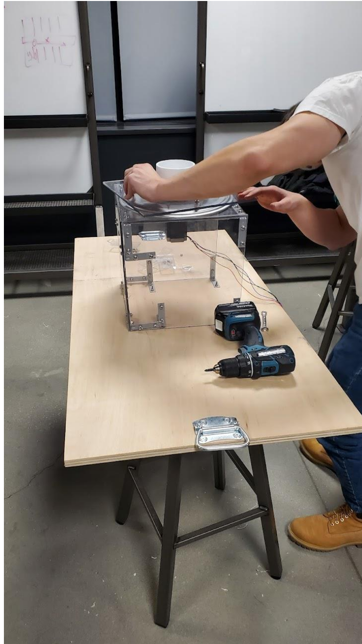
Figure 49: Construction of the Base Station
