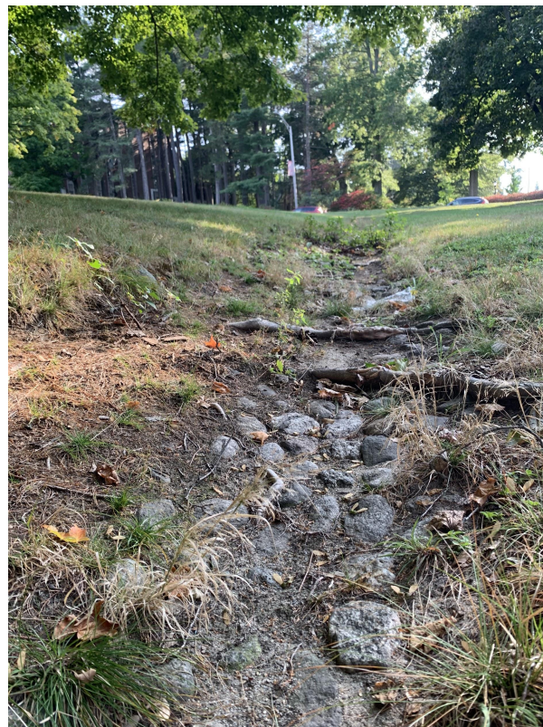
Figure 14-7: Rock and Root Ditch with 1 ½” Bumps
