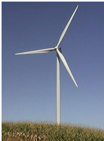
Figure 13: An Example of a Wind Turbine
