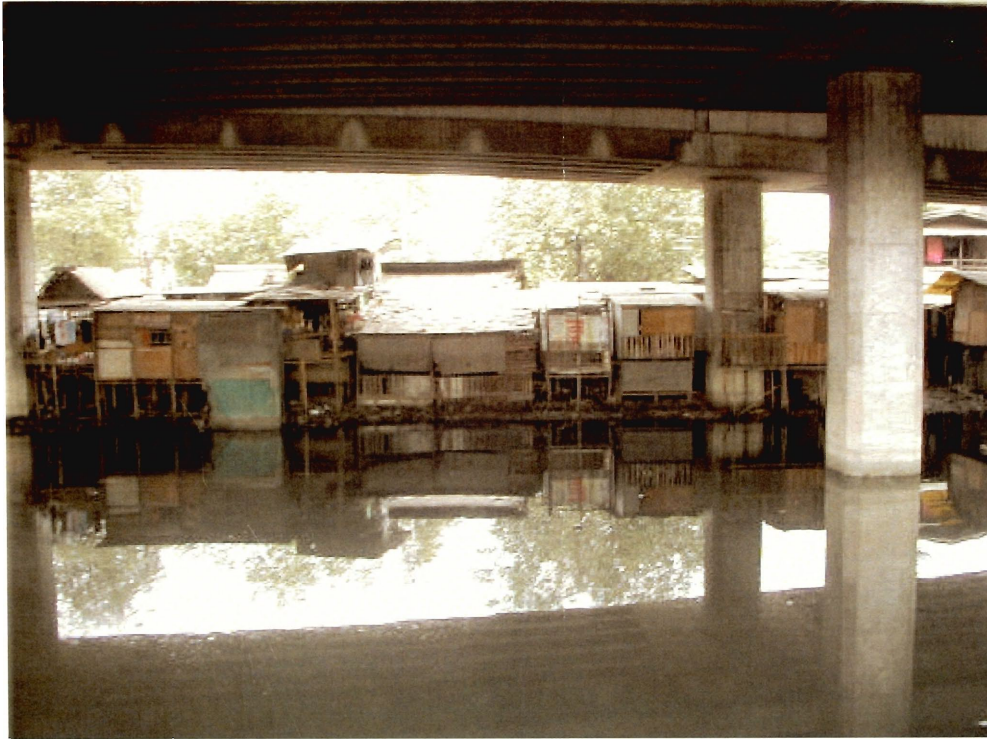
Figure 2: A part of Klong Toey built under the highway
