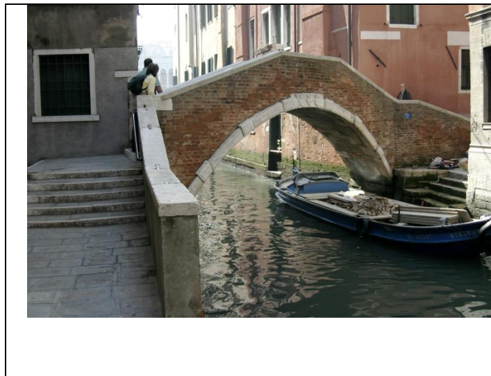
Figure 21 - An example of a pontestorto or "crooked bridge."
