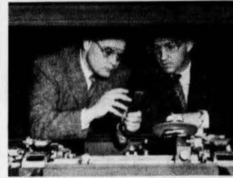
Examining the plastic molded "comb" components of the wire spring relay Dick recalls his early work when he was involved in working-up forming and coining tools for the pilot model of the automation line for fabrication of wire spring sub-assemblies for relays. At present he is associated with the expansion of these automation lines at the Montgomery Plant.
