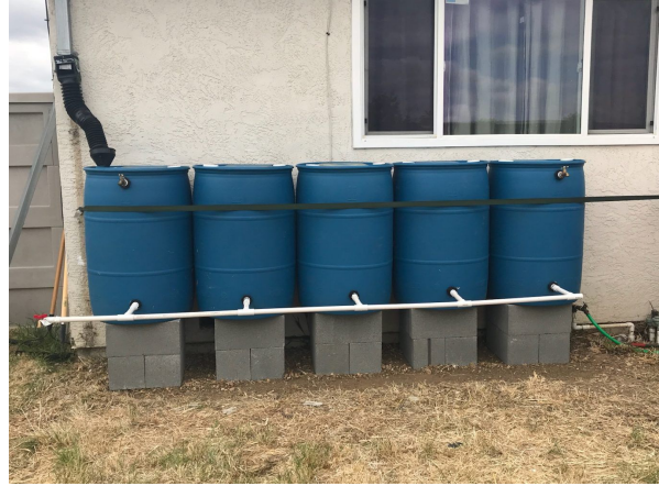
Figure 07: Multi-Barrel System Image Source: Solano, 2018
