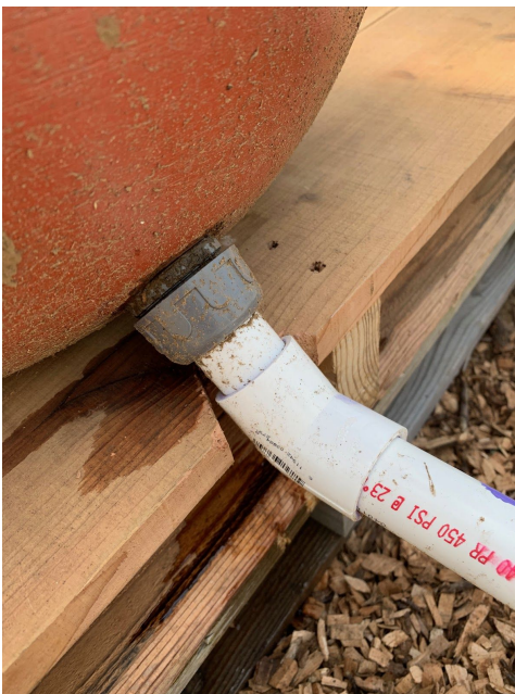
Modification of the wooden pallet to fit the PVC pipe
