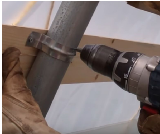
Figure 17: Conduit Strap Installation Image Source: Iowa State University Extension and Outreach Youtube Channel, 2013
