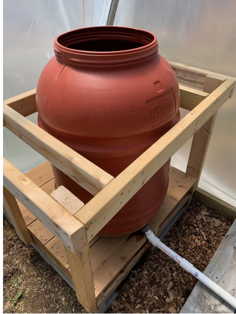
Box made to hold the barrel in place
