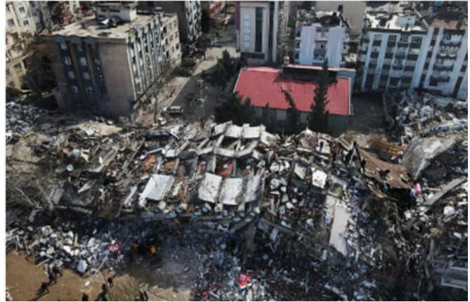
Figure 2: Damage caused by an earthquake in Turkey (Rafferty, 2024).
