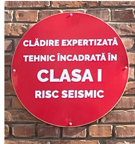
Figure 13: The red circular sign posted on buildings of class 1 seismic risk.
