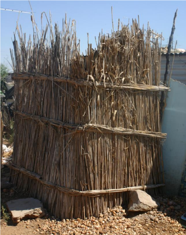
Figure 19: Shower stall made from Reeds in the informal settlements
