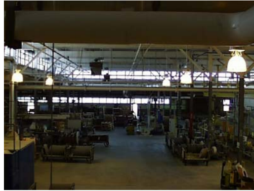
Figure 5.A.1: A snapshot of Plant 7, Norton Co., Worcester, MA.
