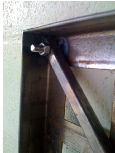
Figure 5- Detail of threaded stud
