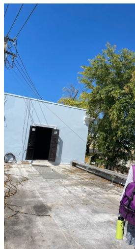
Figure 6: Current Conditions of the Rooftop Space
