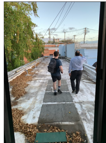
Figure 57: The Vice Mayor Walking Around the Roof
