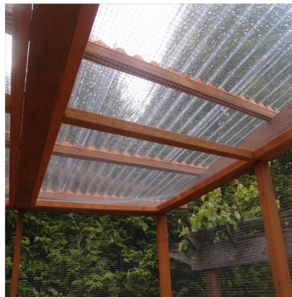
Figure 42: Example of Clear Plastic Sink Ceiling
