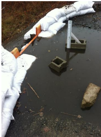
Figure 4: Weir with first water overflow
