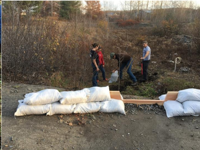
Figure 6: Setup of sandbags at weir
