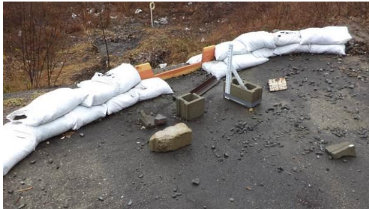
Photo 1: Weir Ready for Storm
