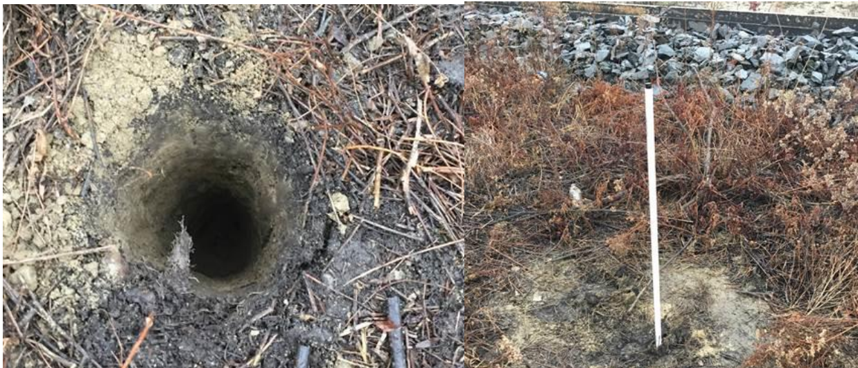
Photo 2: 2' Hole for Groundwater Well
