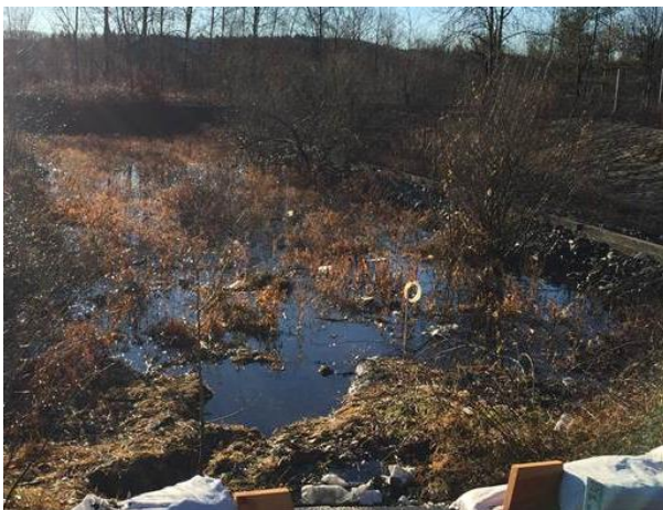
Figure 3: Pooling Water in Chamber 1 (NorthWest View)
