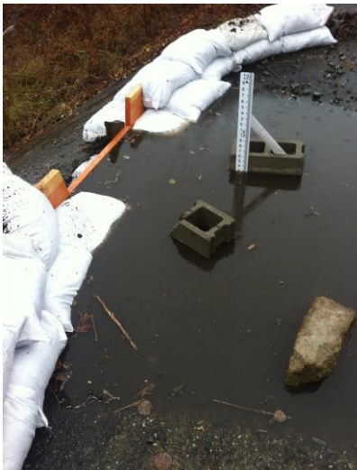
FIGURE 12: STORM RUNOFF POOL
