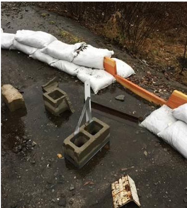
Photo 4: Waiting for the Pool to Fill
