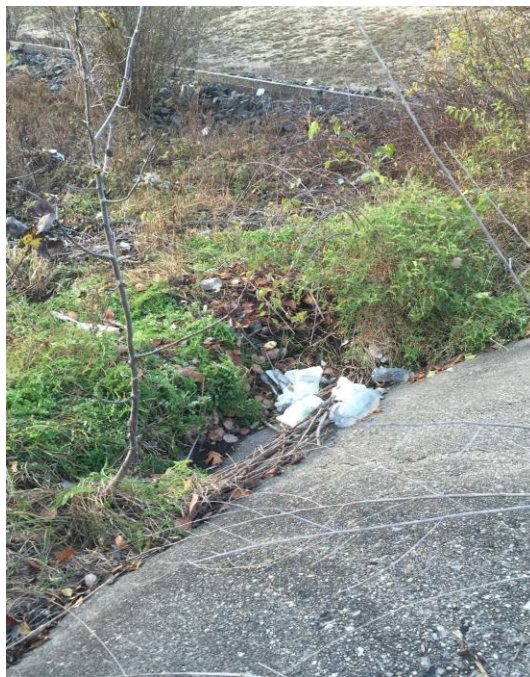
Figure 1: Sediment Build Up
