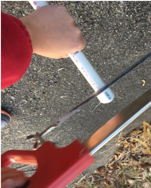
FIGURE 13: CUTTING PIEZOMETER SLITS
