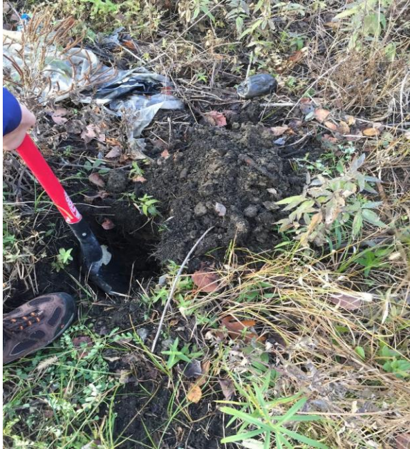
Figure 2: Removing Topsoil with Shovel
