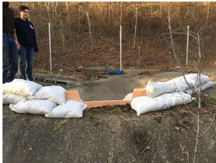
Figure 7: Completed setup of weir and sandbags
