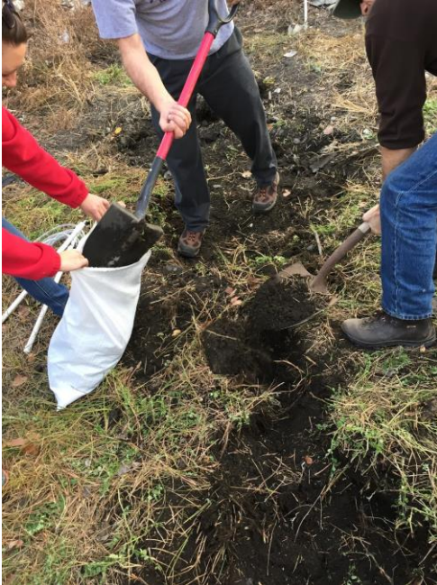
Figure 5: Filling of the sandbags
