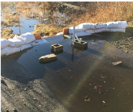
Figure 1: Pool Behind Constructed Weir
