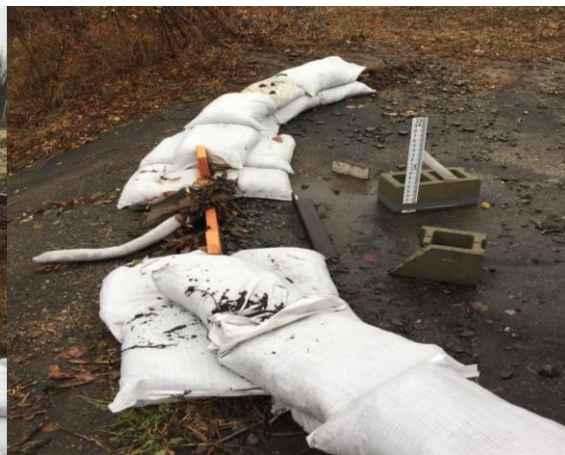
Figure 4: Damaged Weir
