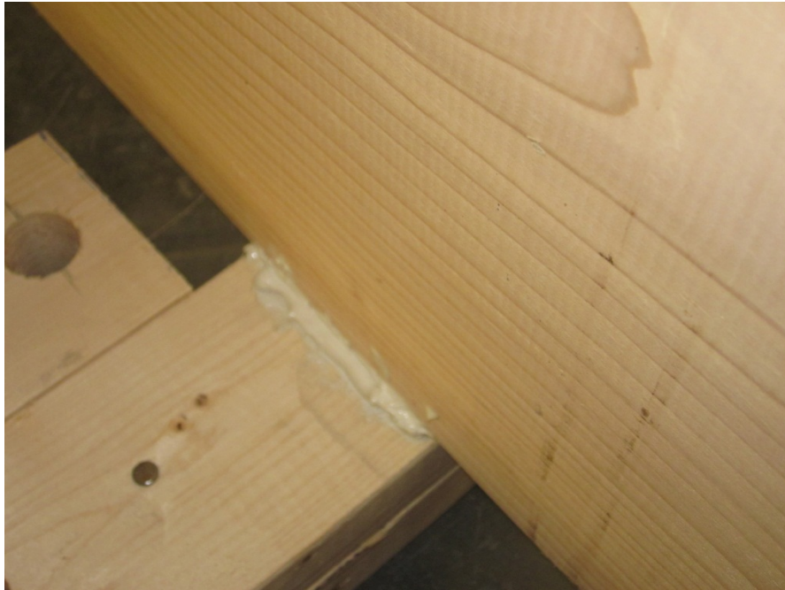
Figure 119: Liquid Nail Connection Specimen
