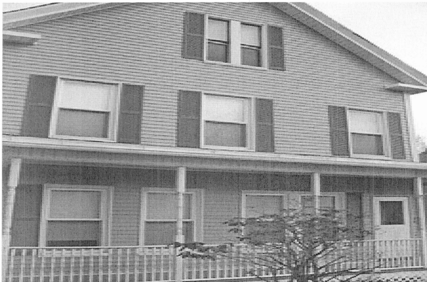
Figure 13. Building with a rating of best.
