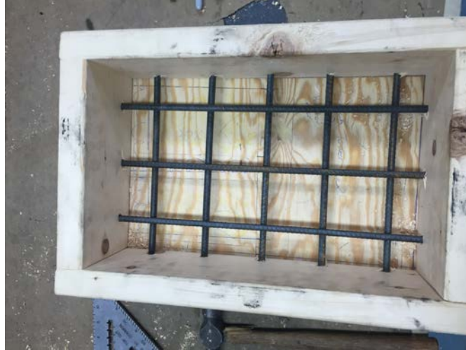
Figure 13: Rebar placement in panel experiment
