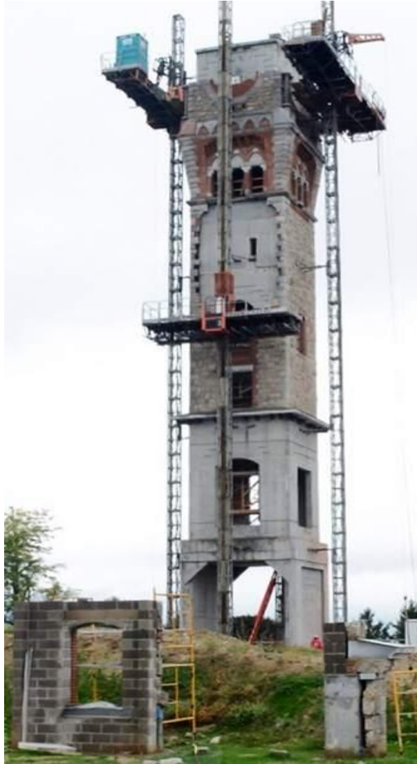
Figure 5: Gilbane's progress of Construction on the Tower
