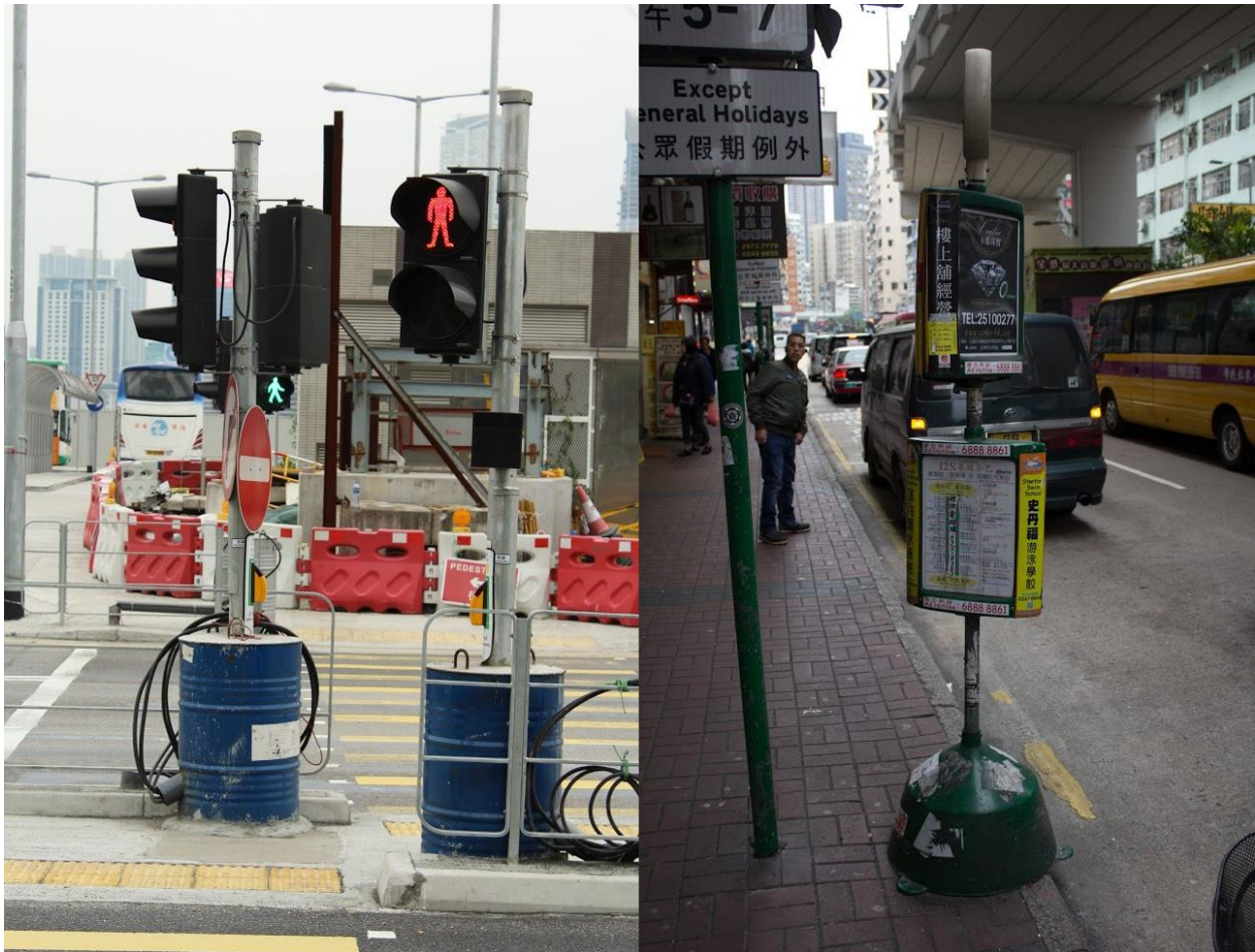
Figure 5.1: Examples of mobile sign posts. On the left is a drum filled with concrete to support a traffic light in a construction site and on the right is a mini bus signpost
