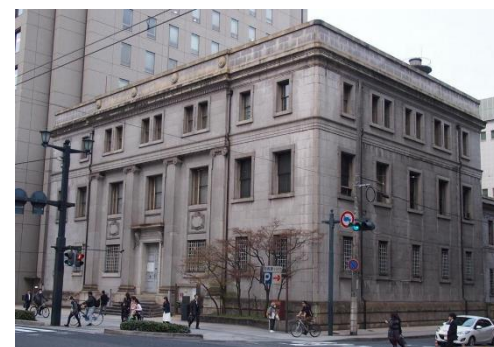
Figure 53. Former Bank of Japan Hiroshima Branch Museum
