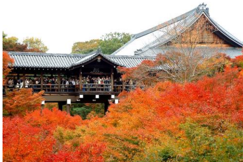
Figure 23. The main building at Tofukuji
