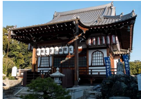
Figure 62: The main building of Myojoin
