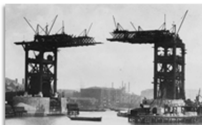
Figure 2: Constructing Tower Bridge
