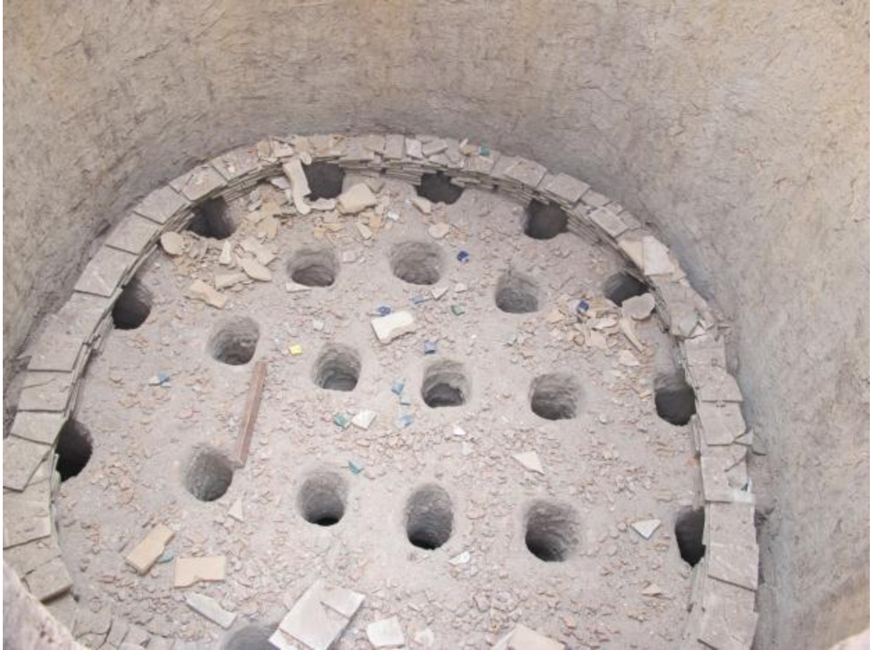
Figure 7: The bottom of the baking chamber of the kiln. The vents allow heat and smoke to enter from the combustion chamber.
