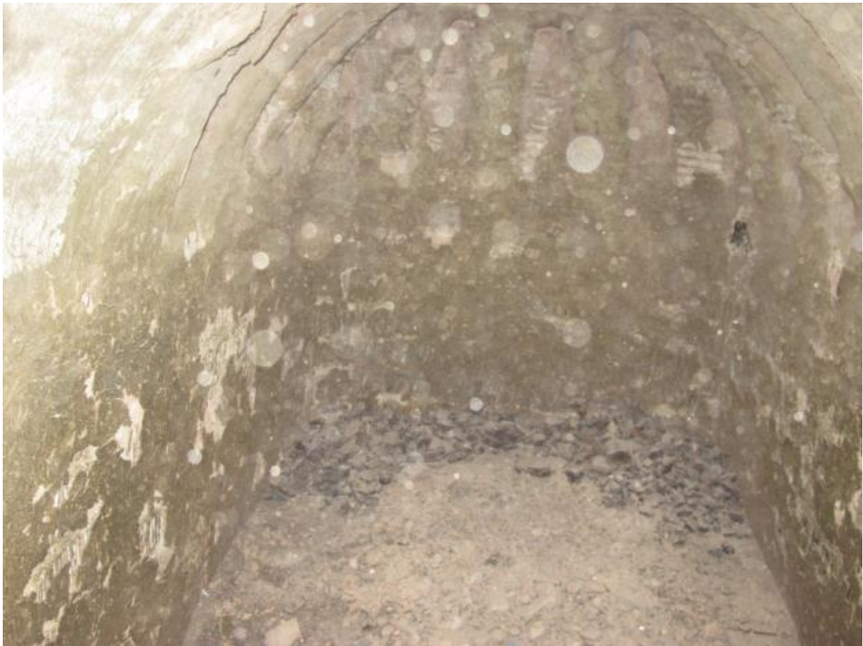
Figure 6: The combustion chamber of the kiln. Note that it is not covered in soot; the kiln is thoroughly cleaned after each use.
