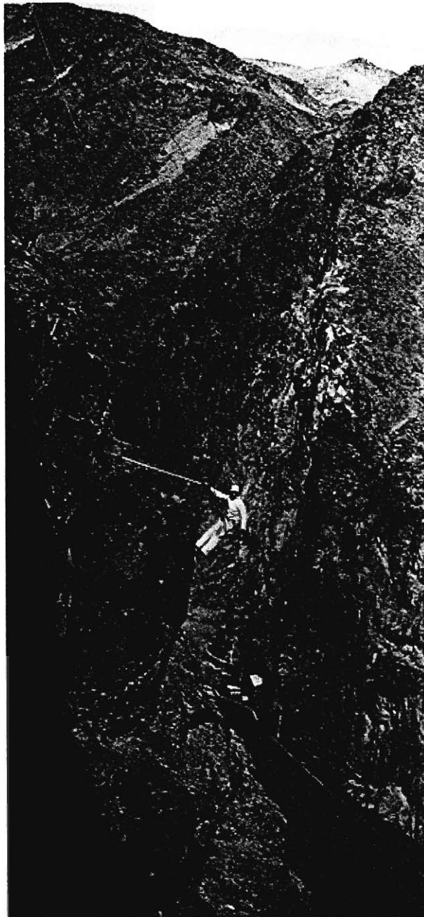
Figure 8: Wall scalers worked to remove loose rocks from the canyon walls that might fall once dam construction began. ( The Grand Colorado: The Story of a River and Its Canyons , p.184)
