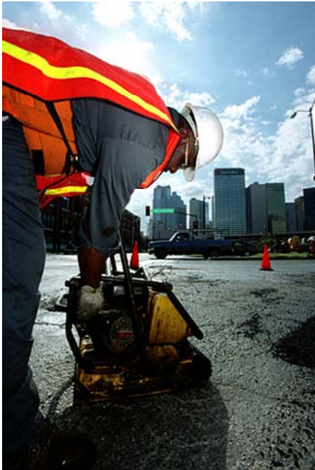
Figure 11 - Fixing Potholes
