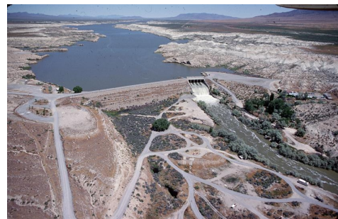
Figure 9.2: Rye Patch Dam and Reservoir
