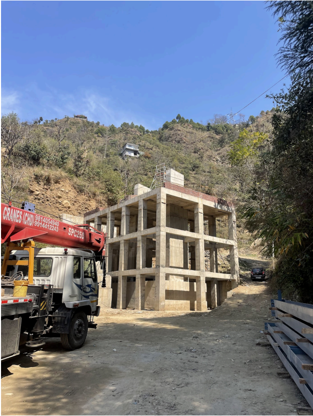
Under construction Baglamukhi top station
