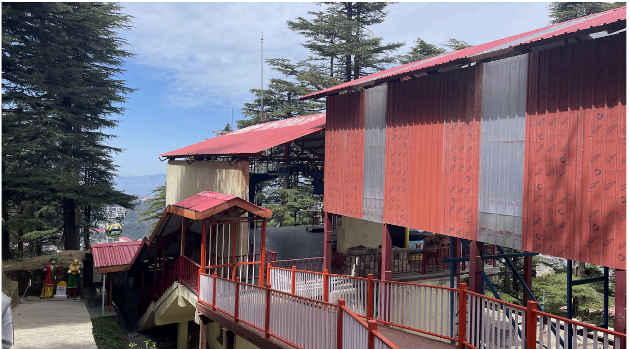
Top station of Jakhu ropeway
