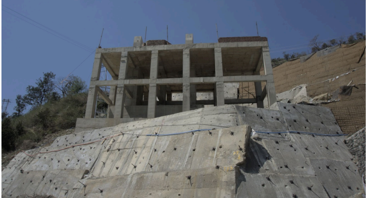
Figure 12: Under construction base station of Baglamukhi Ropeway in Pandali (2024)
