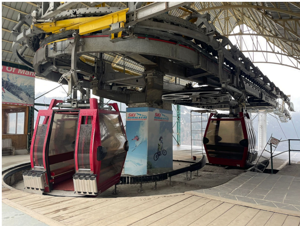
Figure 2: Existing monocable detachable system end station in Manali. One car (Left) in loading mode with doors open and one car (Right) accelerating out of the station onto the moving cable.
