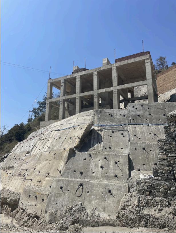
Under construction Baglamukhi bottom station
