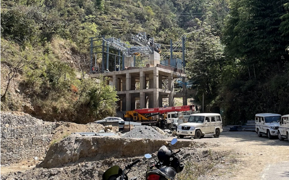
The partially completed top station with initial mechanical system installation underway
