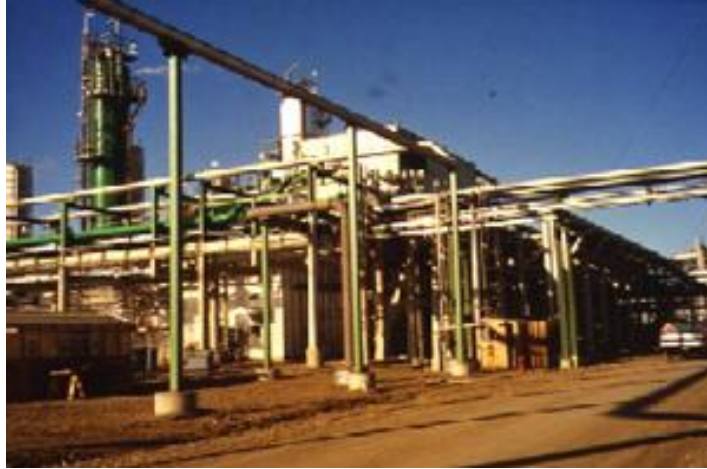
Figure 1: Natural Gas Plant Taken from ( http://www.naturalgas.org/naturalgas/processing_ng.asp )
