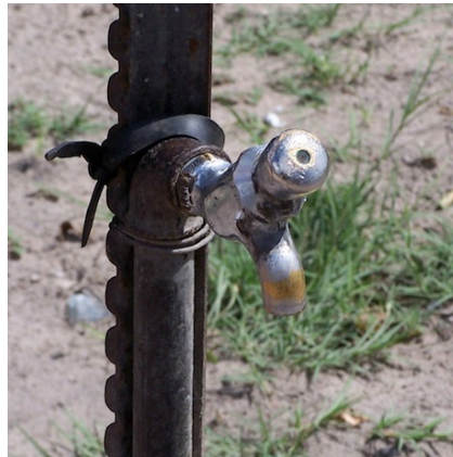
Figure 2.4: This self-closing tap opens only when the button is depressed, preventing it from being left open and forgotten
