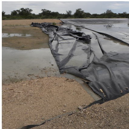
(a) Damage to the oxidation pond lining increases the risk of groundwater contamination
