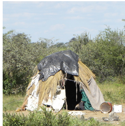
(b) The owner of this hut has incorporated a piece of the lining as rainproofing
