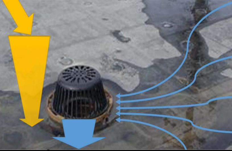
Water from impervious surfaces is directed to combined sewer system
