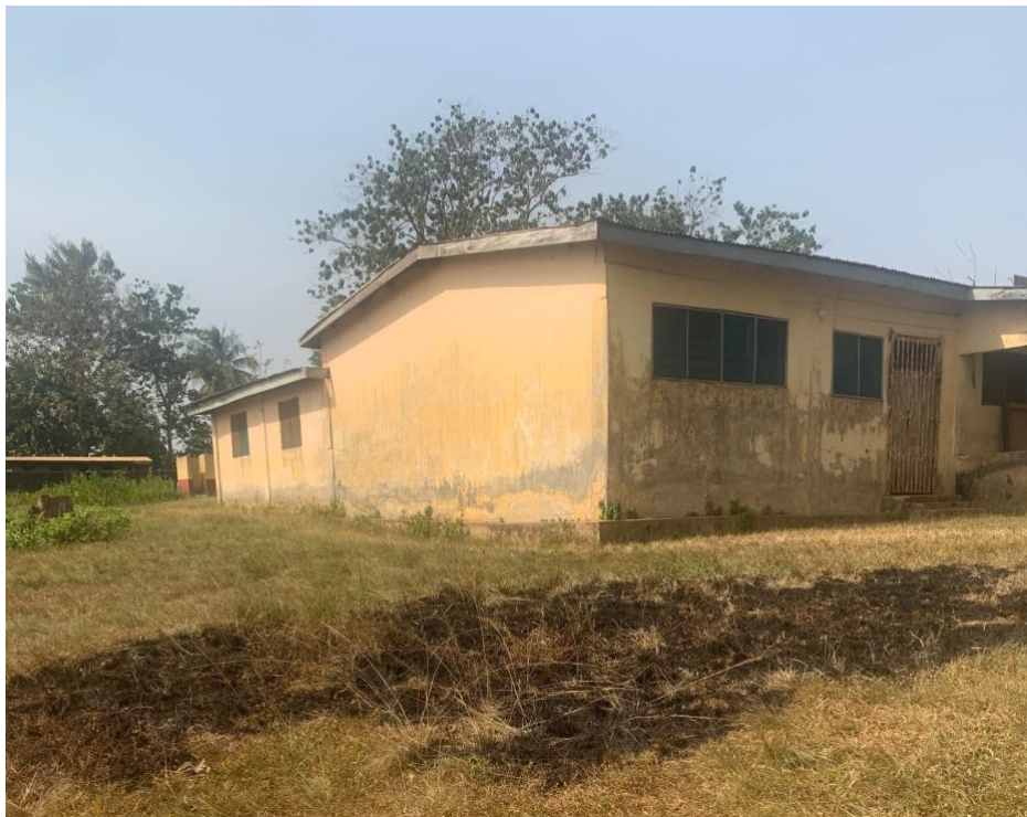
Image: Building which will become the collection center in Akyem Dwenase
