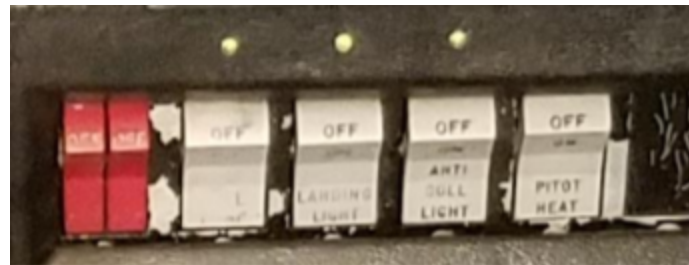
Figure B17: LEDs over Master Switch panel
