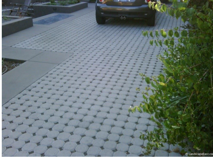
Figure 25. Example of stone pavers with space for water permeation (Stewart, 2017)
