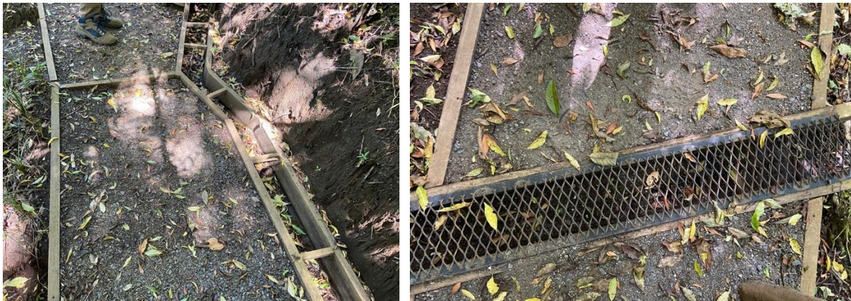
Figures 15 and 16. Design option with gravel and wood siding, with metal grates for drainage
