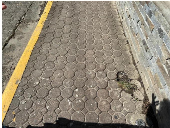
Figure 9. Stone paver sidewalk in downtown Santa Elena.
