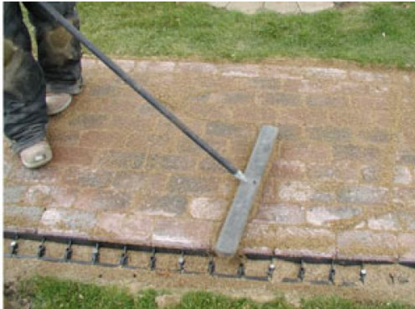
Figure 20: Application of joint sand to installed pavers (Willow Creek, n.d.)
