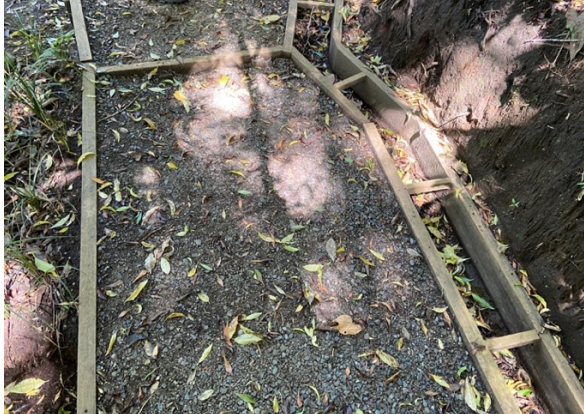
This sidewalk uses materials that can be found locally and has drainage channels.
