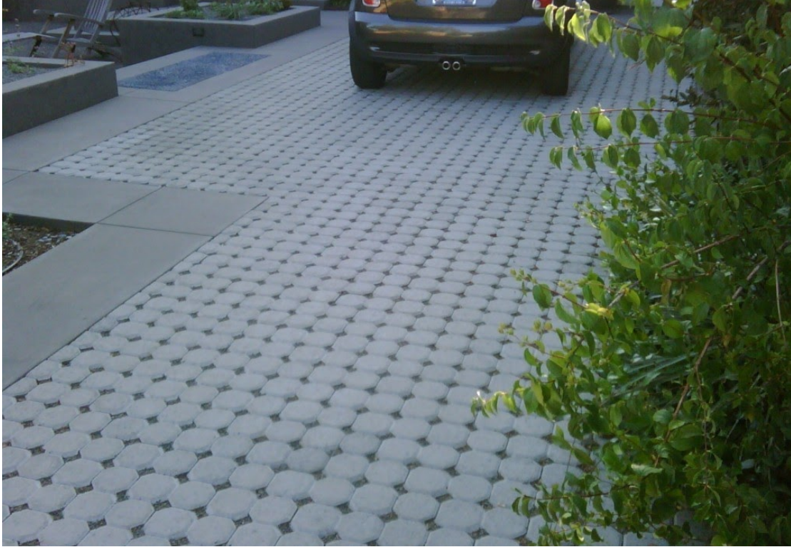
Figure 23: Example of permeable stone pavers (Stewart, 2017).
