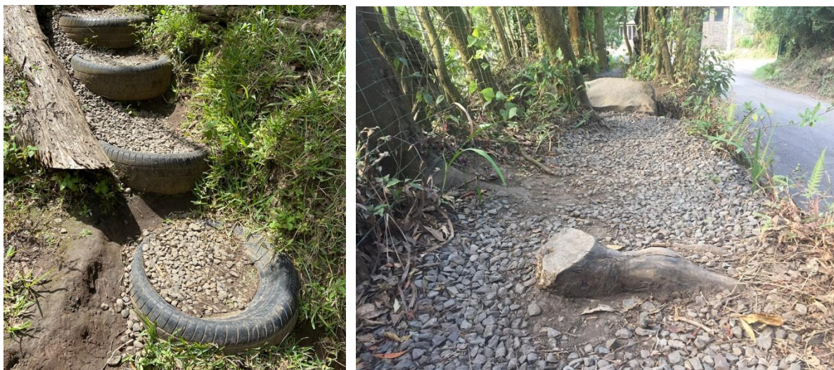
Figures 7 and 8. Example of a location where a raised sidewalk has been implemented with alternative stairs.
