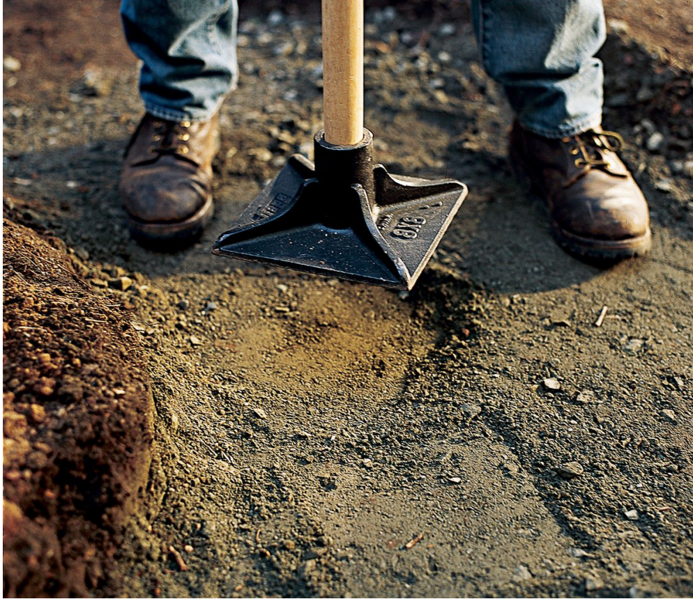
Figure 28: Compacted subgrade stone layer (Bandon, 2007).
