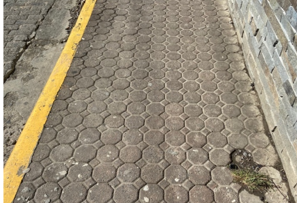
Stone or brick pavers can be used to construct a sidewalk that is non-slip, easily accessible, and can drain to the road easily.
