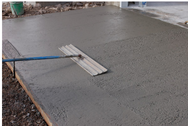
Figure 9: Concrete float being used to smooth concrete (Suryakanta, 2014).
