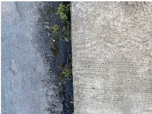
This concrete is corrugated to prevent slipping and has a drainage ditch on the side to prevent water pooling.
