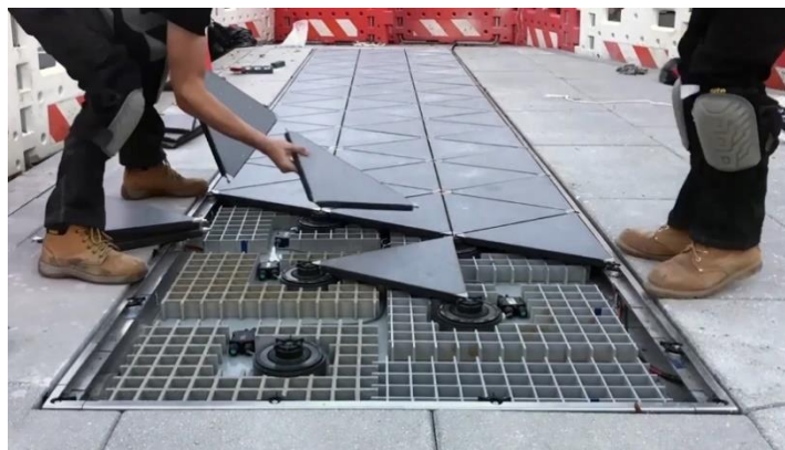
Figure 4. PAVEGEN energy absorbing sidewalk (PAVEGEN, 2019).
