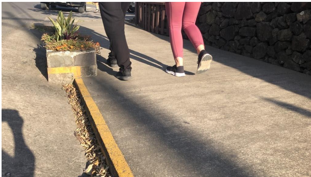
Figure 12. Concrete sidewalk near Poco a Poco, Monteverde.
