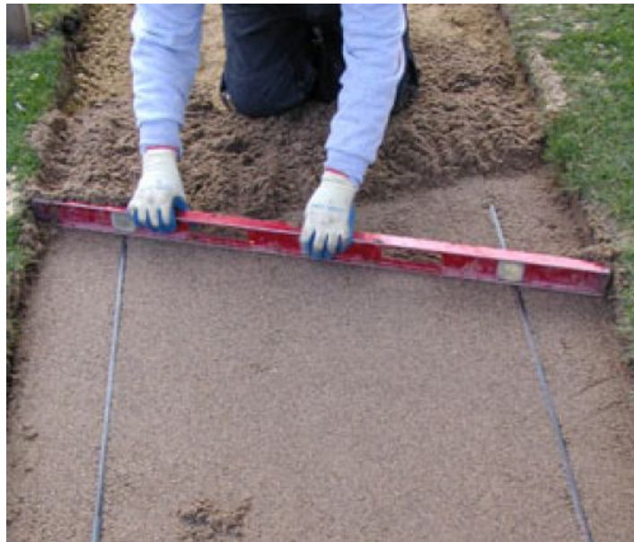
Figure 19: Screed rails used in paver installation (Willow Creek, n.d.)
