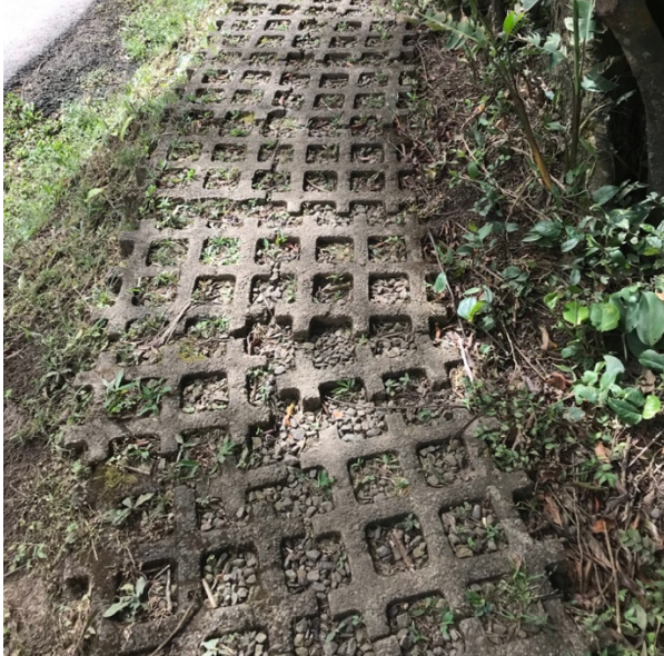
Waffle pattern sidewalks can catch people’s feet as they’re walking, causing them to trip and fall
