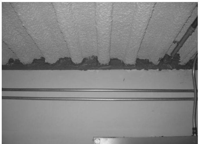
Figure 107 Illustration of Vertical Continuity of Fire Barriers
