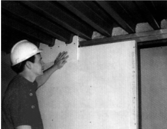
Figure 28 Illustration of Vertical Continuity of Fire Barriers (Puchovsky, 2009)
