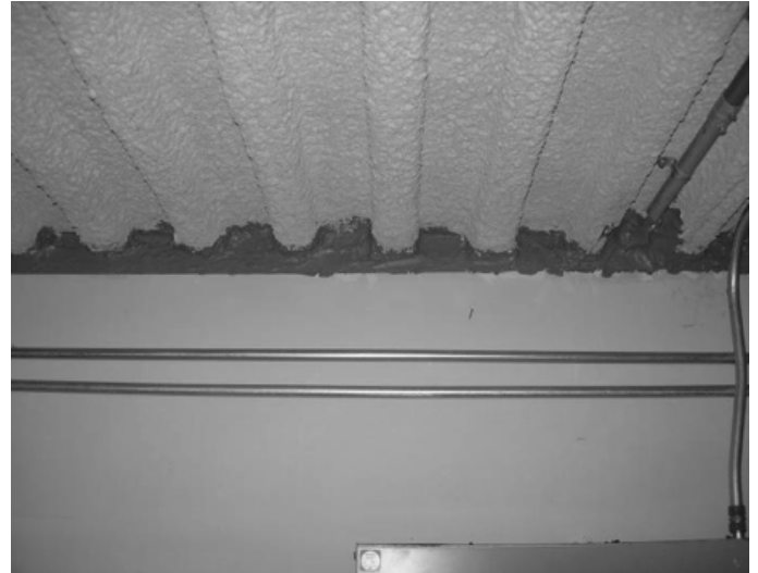
Figure 28 Illustration of Vertical Continuity of Fire Barriers (Puchovsky, 2009)
