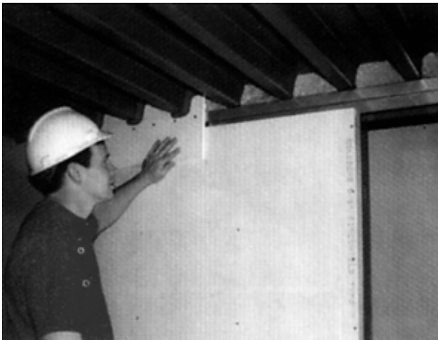
Figure 107 Illustration of Vertical Continuity of Fire Barriers
