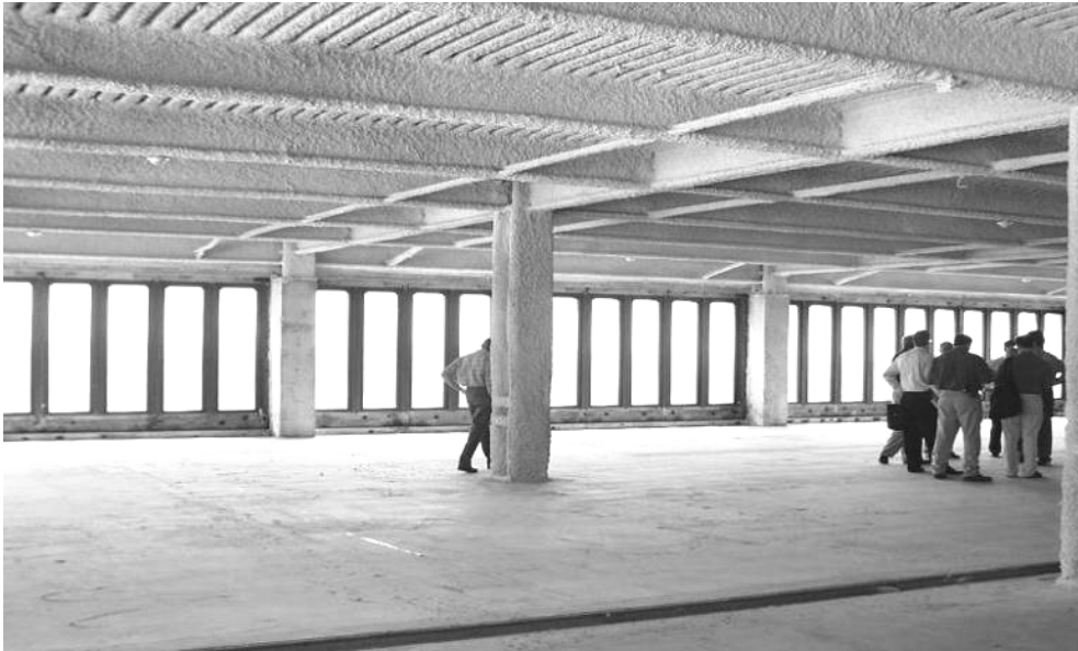
Figure 89 Type II with Protection ( FP570-module 7)
