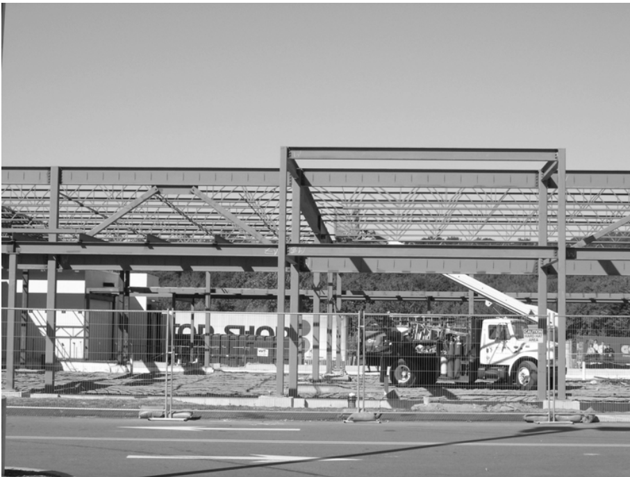
Figure 90 Type II without Protection ( FP570-module 7)
