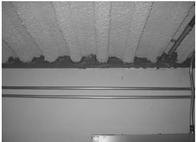
Figure 96 Illustration of Vertical Continuity of Fire Barriers
