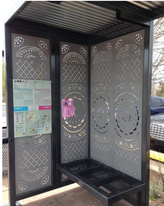
Figure 8: New Bus Stops with Route and Schedule Display
