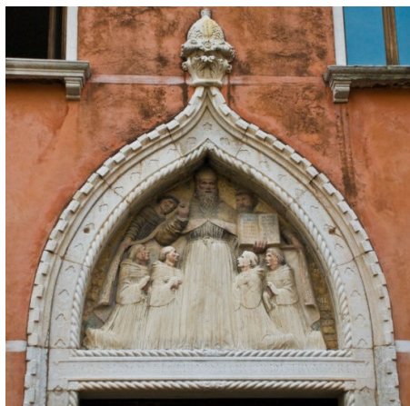
Figure 46: A gothic lunetta with paint still present.
