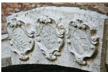
Figure 48: A bridge keystone decorated with three stemmi
