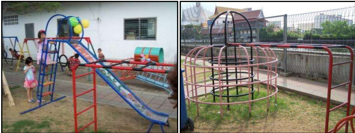
Figure 19. Final positioning of the metal slide (left) and large metal climber (right).
