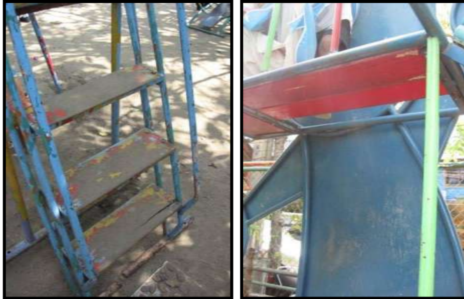
Figure 14. Major safety concerns on the single slide include loose and broken stairs (left) and missing or cracked floorboards on the Mickey slides (right).
