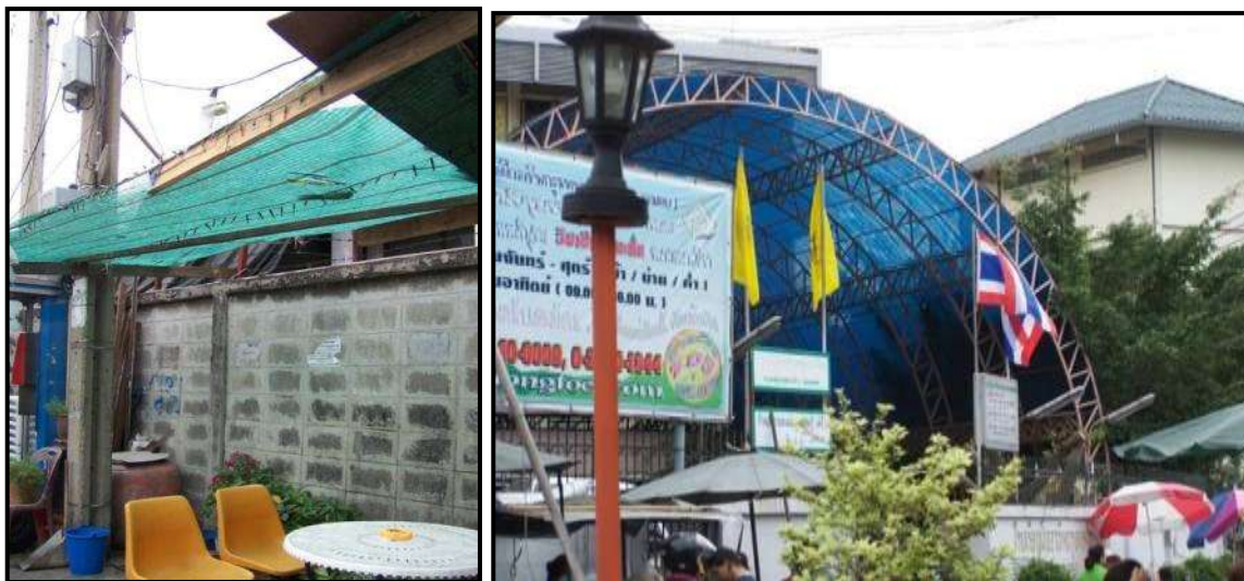
Figure 8. Mesh net (left) and tarp (right) roofs in Klong Toey
