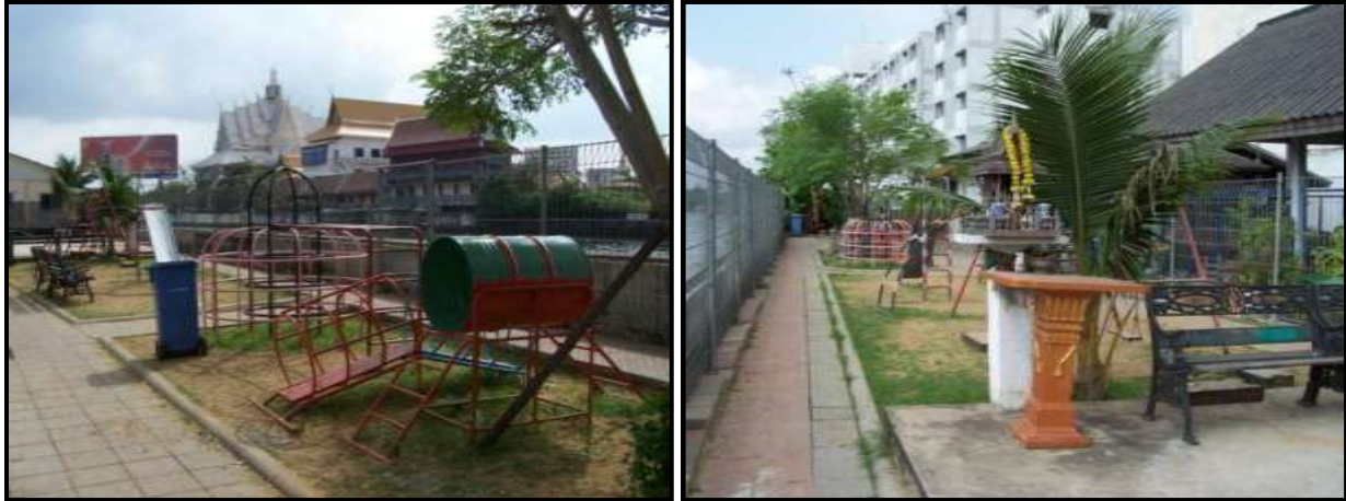
Figure 15. The Lock 23-24 community playground in Klong Toey, Bangkok, prior to its renovation
