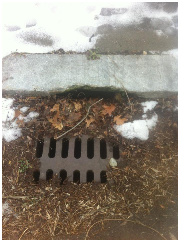
Figure 16 Storm drain with no Stenciling
