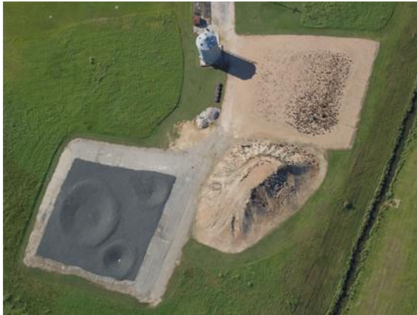
Figure 12: Bird-eye View of JSC's Rock Yard
