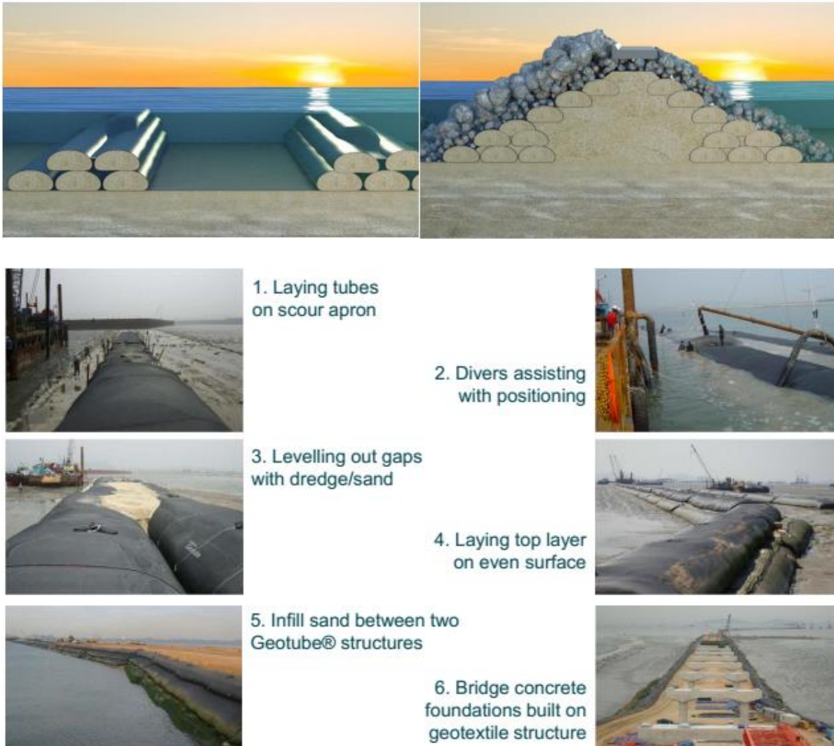
Figure 3.2.29: Construction of bund for tidal lagoon 95
