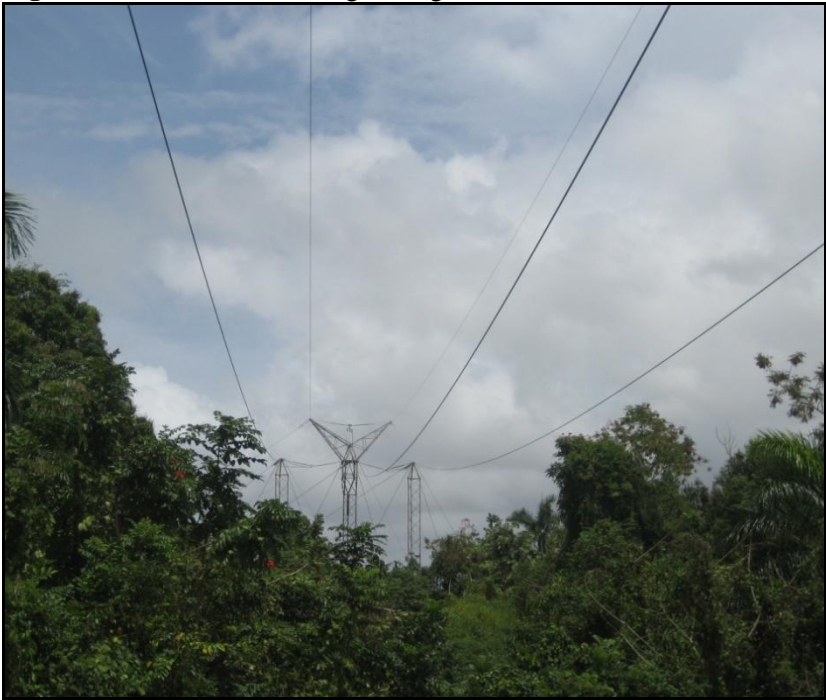
Figure 7: Power lines running through the Conservation Easement.
