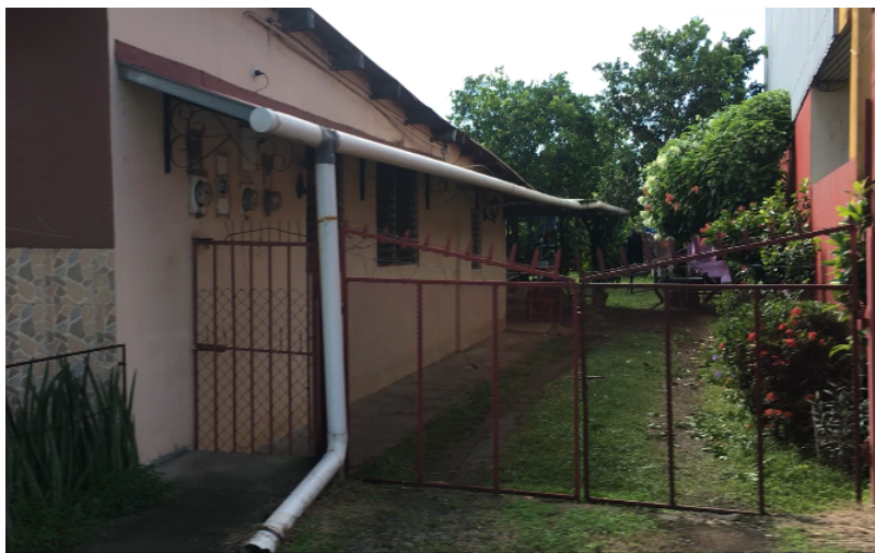
Figure 11: CPVC piping being used as a conveyance system at a household in David
