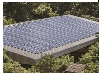
FIGURE 19: EXAMPLE OF ROOF SOLAR ARRAY
